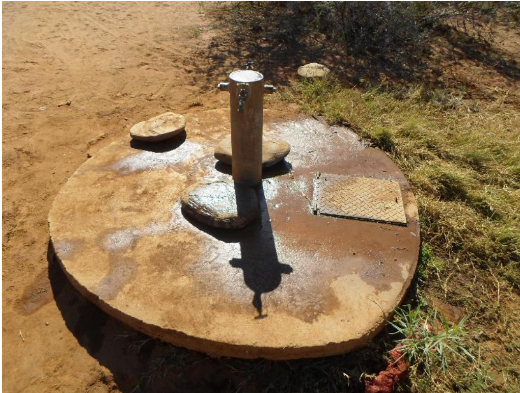
Figure 15: Impacted shared water source
